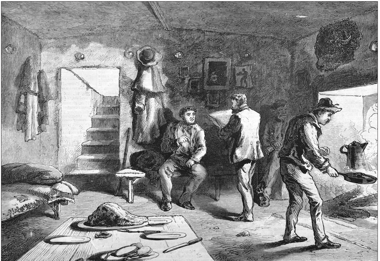
THE FAR WEST. -- INTERIOR COVERING OF A DUG-OUT ON THE LINE OF THE KANSAS PACIFIC RAILWAY.
